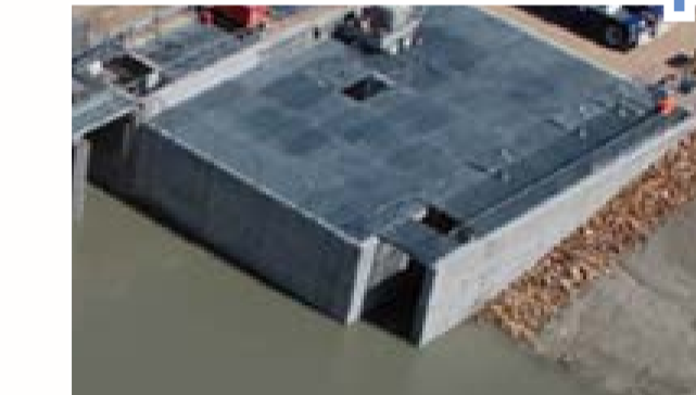
Indicative image of a fishway associated with a very large regulator located to the right
