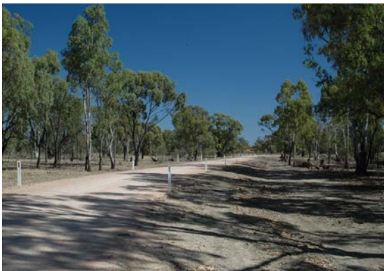
Example of a raised track containment bank at Hattah Lakes
