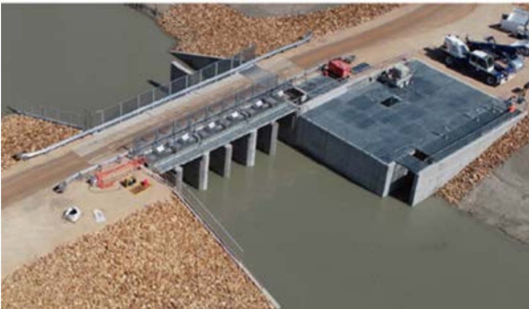
Example of a large regulator at Pike Floodplain in South Australia
