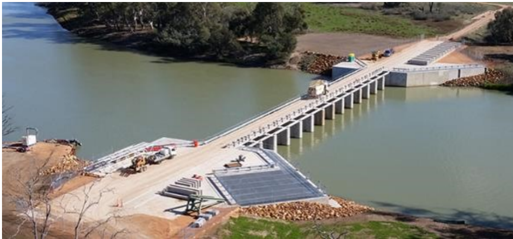
Figure 3: Example of a very large regulator (Chowilla Creek Weir) in South Australia
