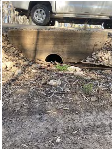
Example of existing infrastructure that blocks the flow of water through the floodplain
